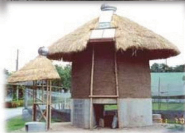
Vetiver clay bundles paddy storage by Nimityongskul and Hengsadeegul et.al. 2004
